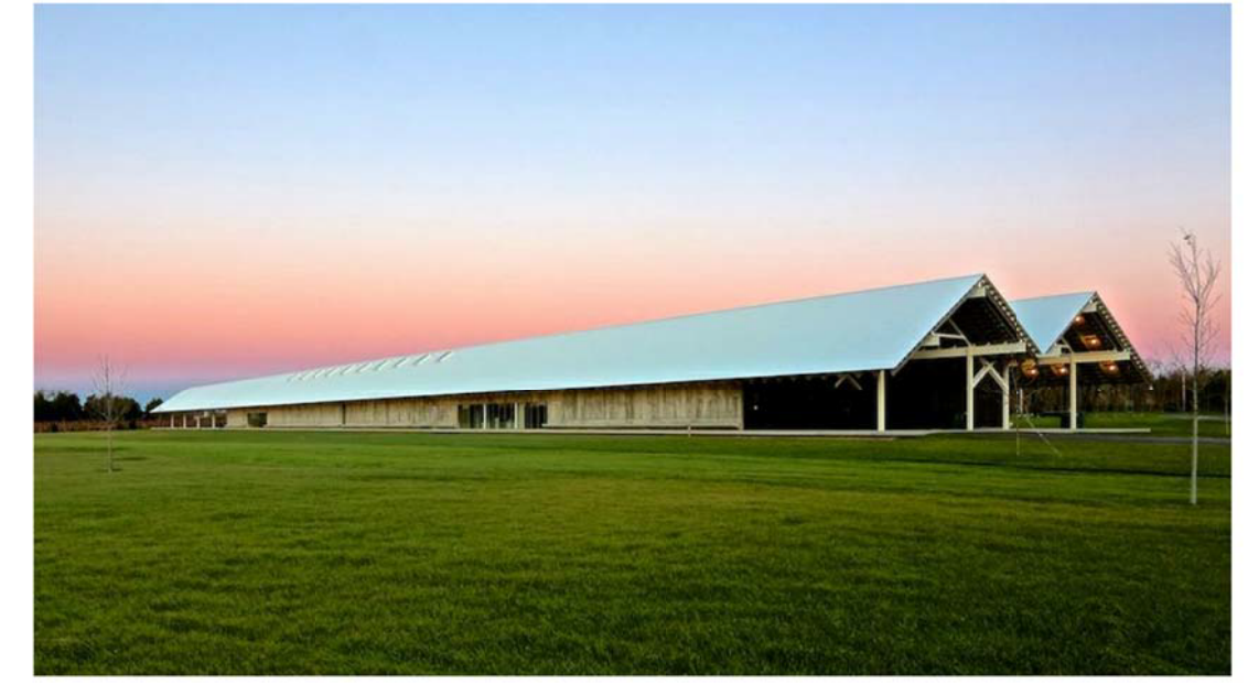
LANDMARK SHED ROOF FORM
